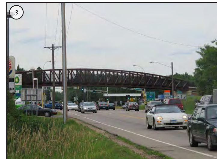
Century Avenue/Division Street and Highway 36 interchange and Gateway Regional Trail
