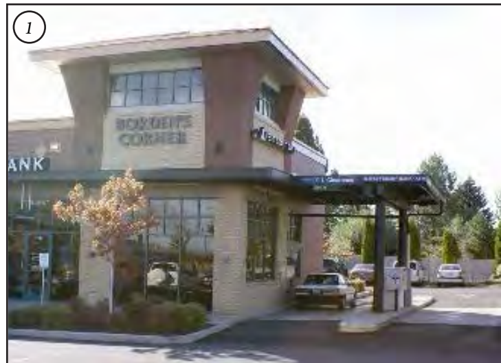
Convenience retail could posses drive-thru on the end caps of in-line retail buildings.
