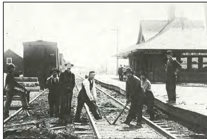
Repairing the tracks at the historic North St. Paul Depot (Image: A Century of Good Living-North St. Paul)
