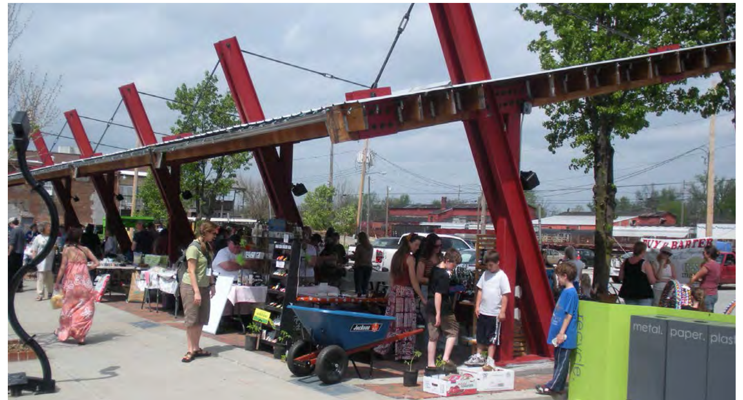
A permanent farmer's market pavilion is envisioned with urban park enhancements and improved parking and visibility to the Library as a part of this phase.
