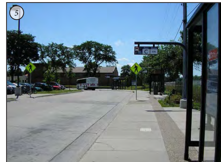
Park and Ride Facility
