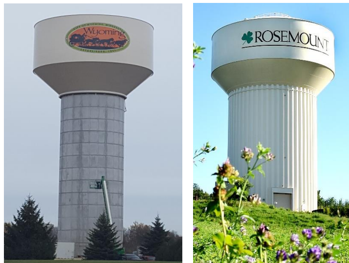
Figure 2. Composite Water Tower (left) and Fluted Water Tower (right)
