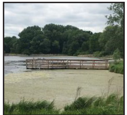
Fishing Pier constructed in 2015
