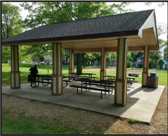
Shelter replaced in 2012
