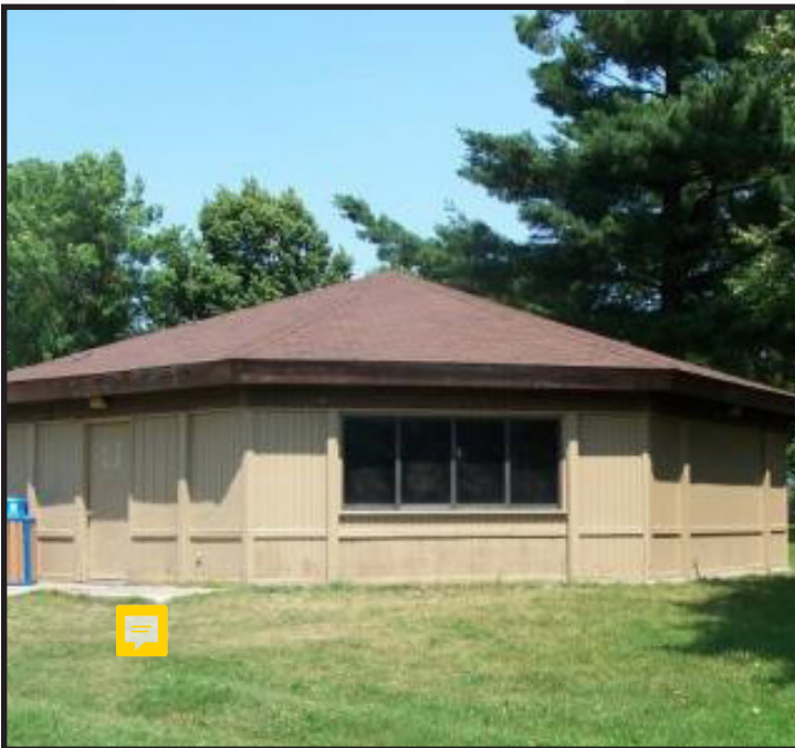
Renovation of the park building 2018
