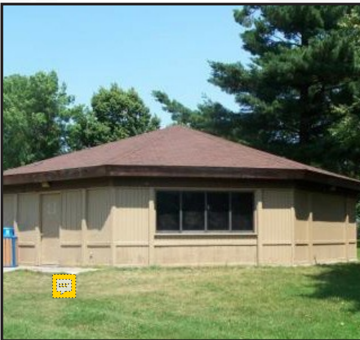
Renovation of the park building 2018
