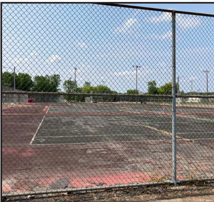
Tennis courts in poor condition
