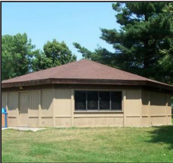
Renovation of the park building 2018
