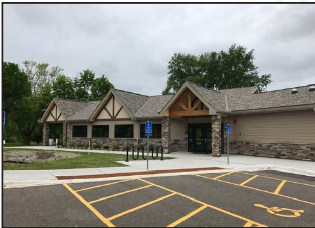
Shelter and park building renovated/ rebuilt in 2016
