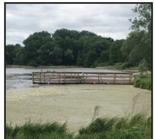
Fishing Pier constructed in 2015
