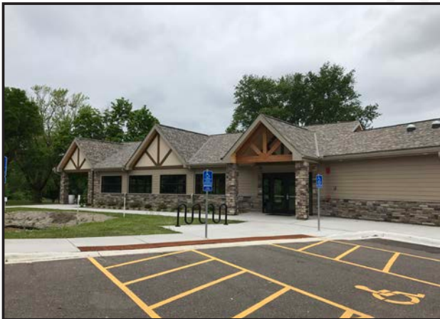
Shelter and park building renovated/ rebuilt in 2016
