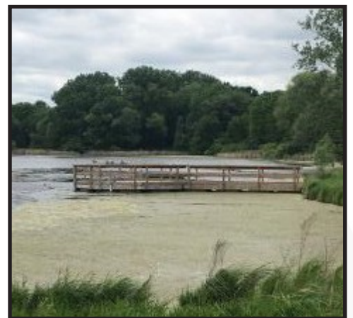
Fishing Pier constructed in 2015
