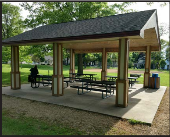
Shelter replaced in 2012
