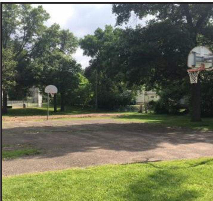
Basketball Court in poor condition
