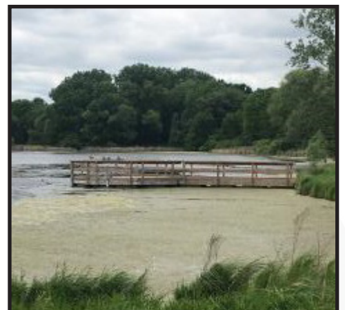
Fishing Pier constructed in 2015
