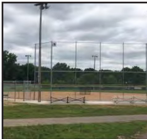
Field #1 renovated in 2017
