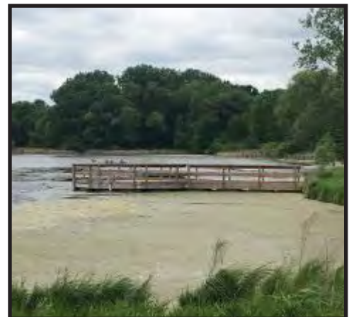
Fishing Pier constructed in 2015
