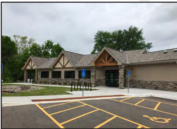
Shelter and park building renovated/ rebuilt in 2016
