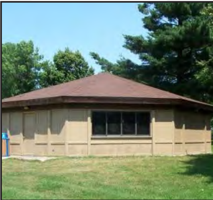
Renovation of the park building 2018
