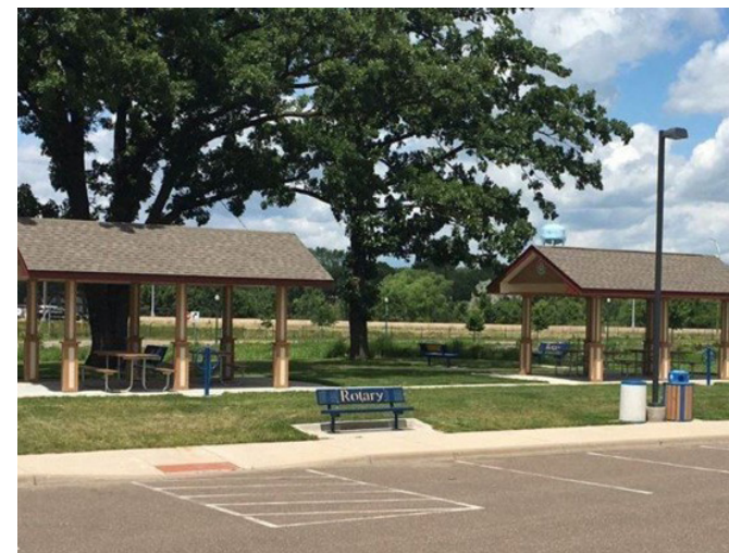
EXISTING ROTARY PARK PAVILIONS
