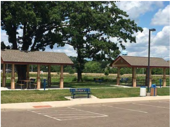
EXISTING ROTARY PARK PAVILIONS
