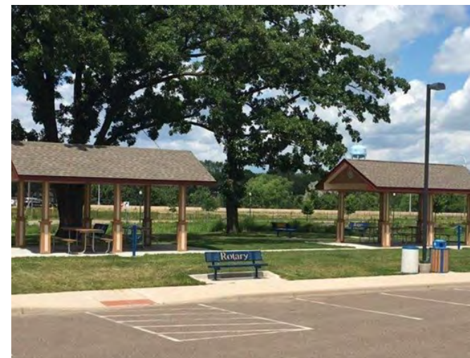
EXISTING ROTARY PARK PAVILIONS
