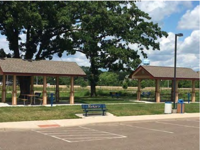
EXISTING ROTARY PARK PAVILIONS
