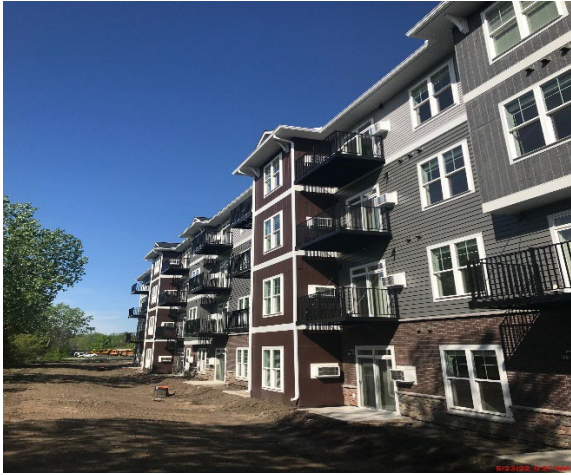
Anchor View Apartments
