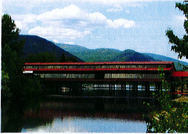
The reconstructed Cedar Street Bridge in Sandpoint, Idaho, is now an enclosed linear retail walkway linking the train depot to downtown businesses.
