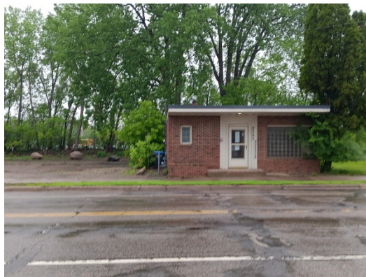
Existing structure at 2393 Margaret Street
