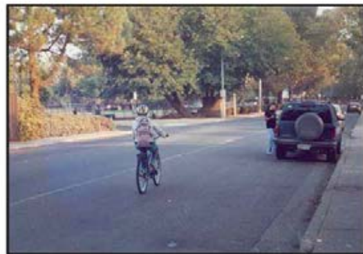
Wide Paved Shoulder
