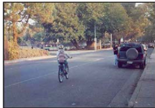
Wide Paved Shoulder
