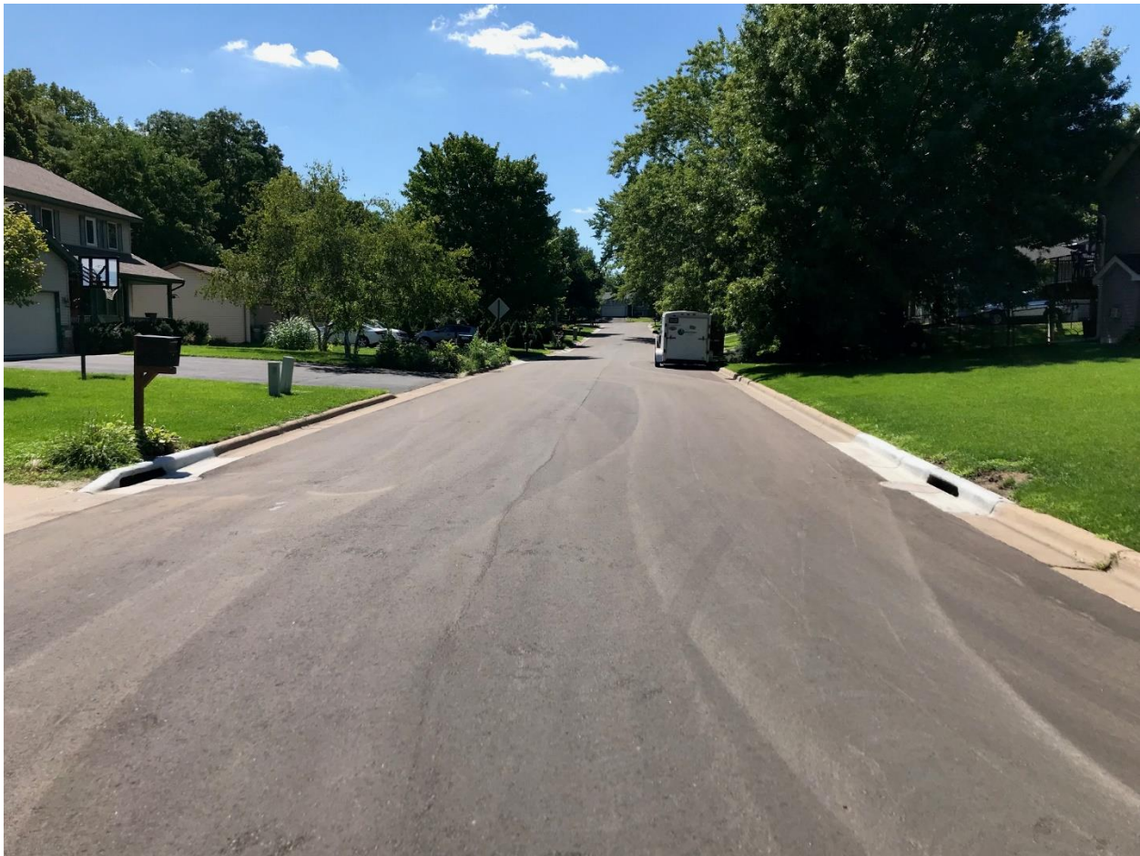
Figure IV.1. Recently Completed Maintenance Overlay
