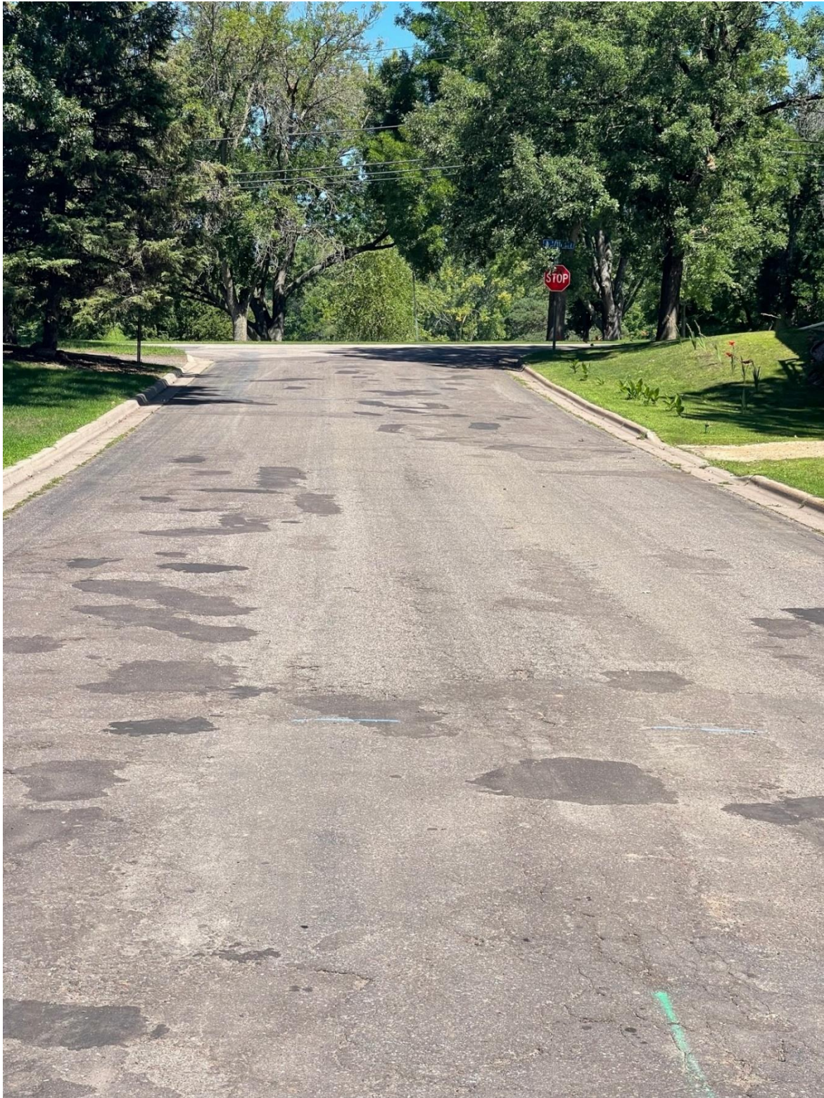
Figure IV.2. Segment That Will Soon Receive a Maintenance Overlay
