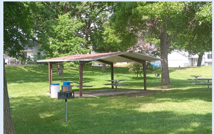
Northwood Park Shelter
