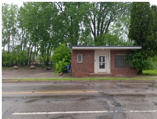
Existing structure at 2393 Margaret Street
