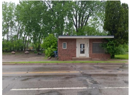
Existing structure at 2393 Margaret Street
