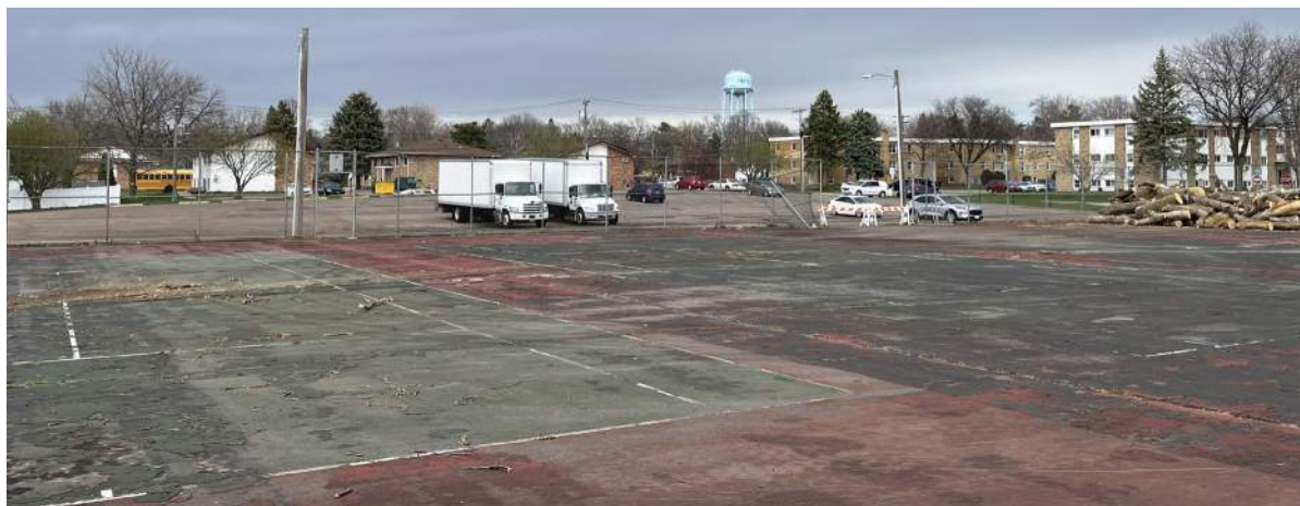
E - Unused tennis courts in disrepair
