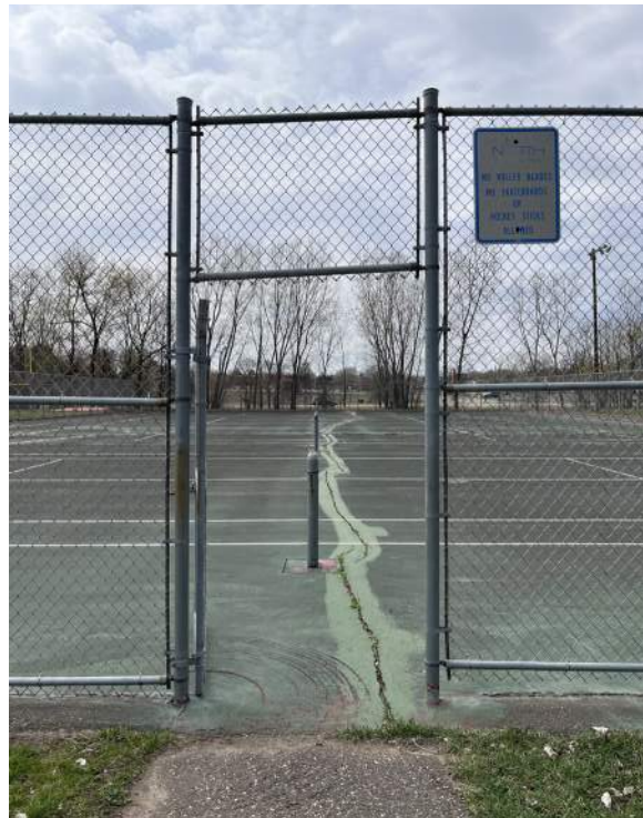
B - Unused tennis courts in disrepair
