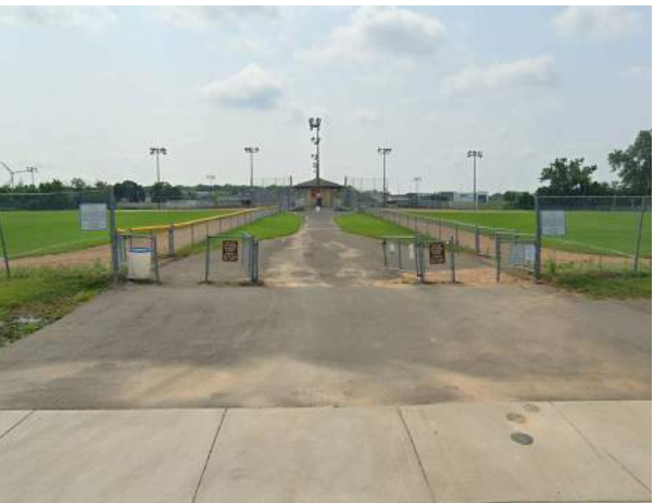
F - Fence, gates and signage restricting access
