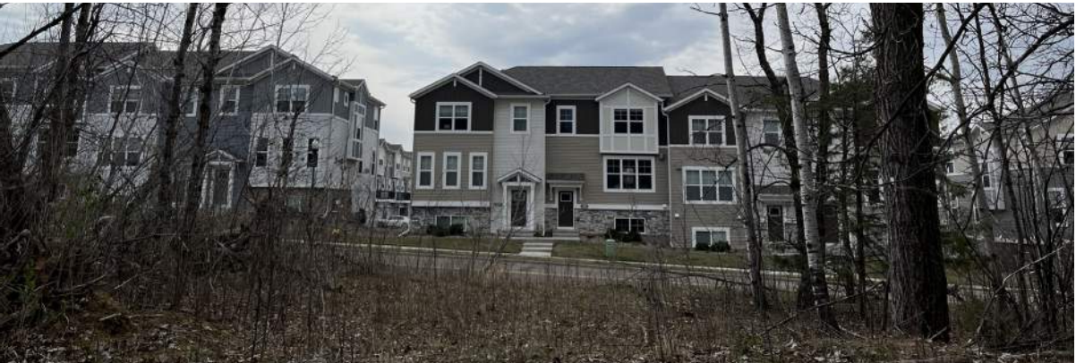
C - Unused tennis courts in disrepair
