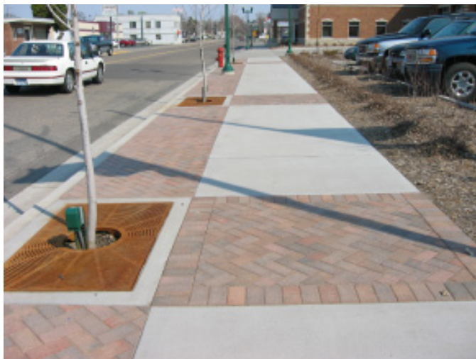
The paving pattern in front of city hall is herringbone with a soldier course perimeter. The pavers are the Holland paver from Anchor Block in the North Oaks color.
