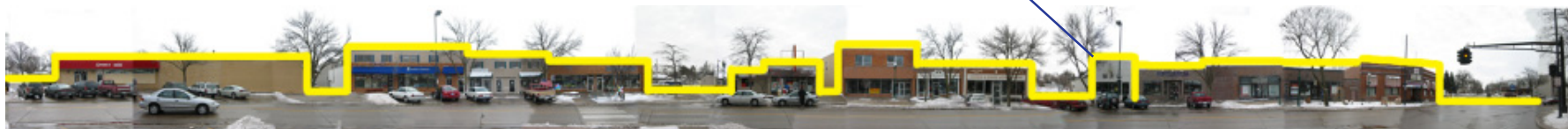
Image below: Southern streetwall of 7th Avenue between Charles and Margaret. Notice the one and two-story buildings, and the parapet on Shangri-La. The parapet increases the effective height of the building.
