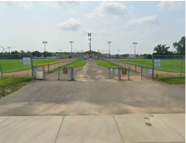
F - Fence, gates and signage restricting access
