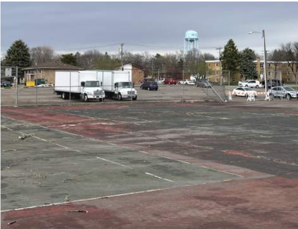
E - Unused tennis courts in disrepair
