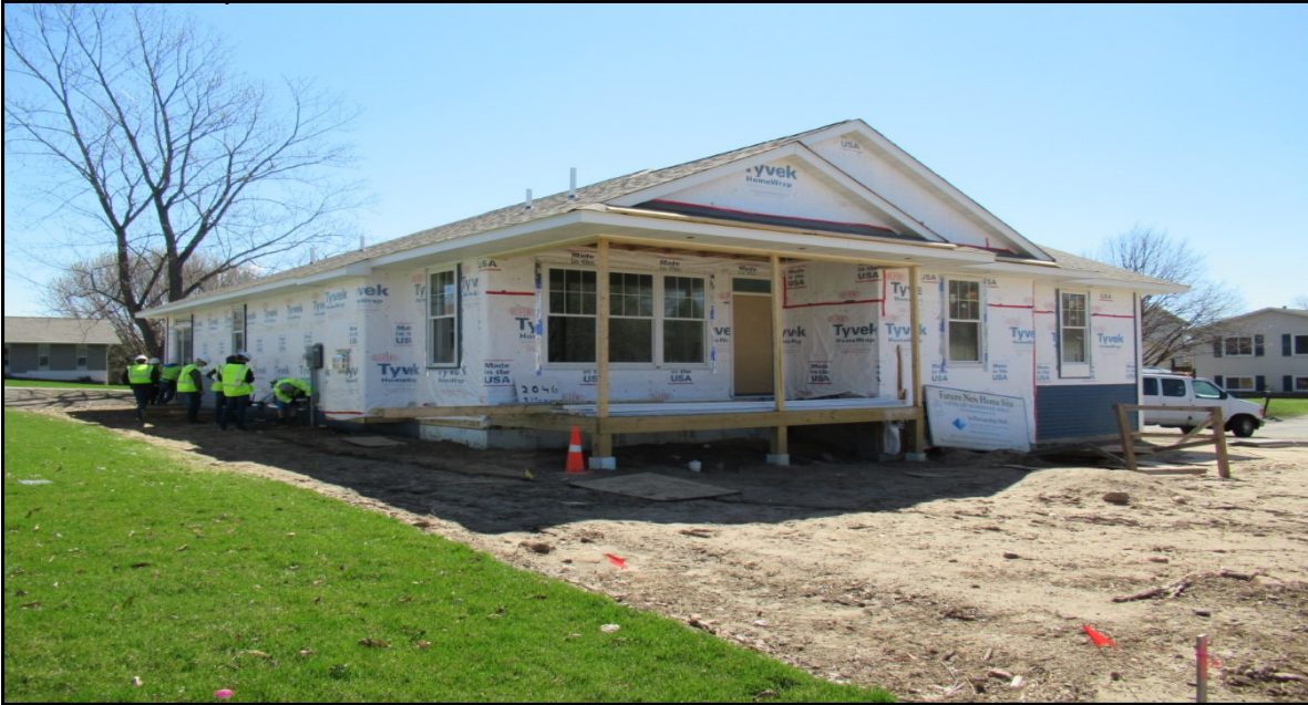
FRONT VIEW OF SUBJECT PROPERTY
