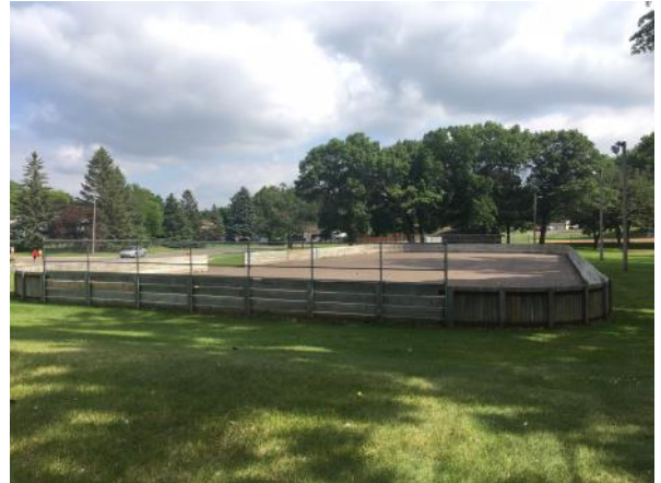
Hockey Rink is in good condition
