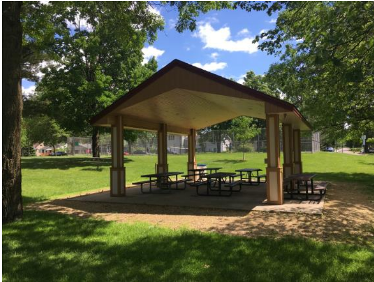
Shelter replaced in 2012
