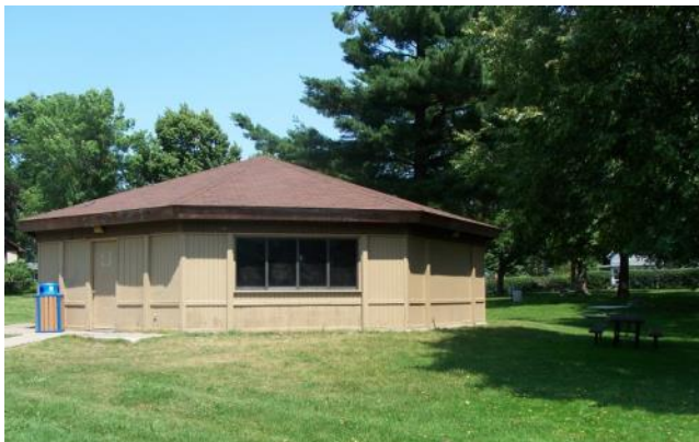
Renovation of the park building completed 2018
