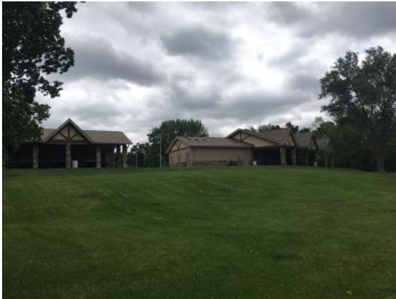
Shelter and park building renovated/rebuilt in 2016
