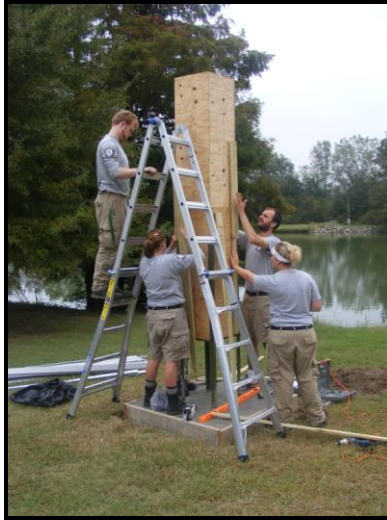
Assembling braces against the edges of two connecting nesting chambers.
