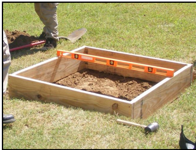
A level foundation formed on an uneven, hilly surface. Notice a bubble level is used to ensure that the entire foundation is level.
