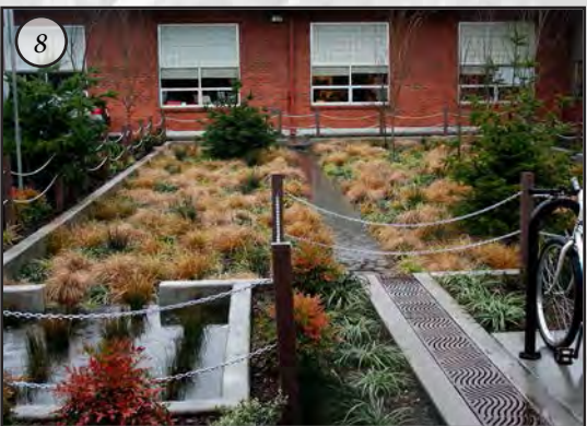
Creative on-site stormwater solutions
