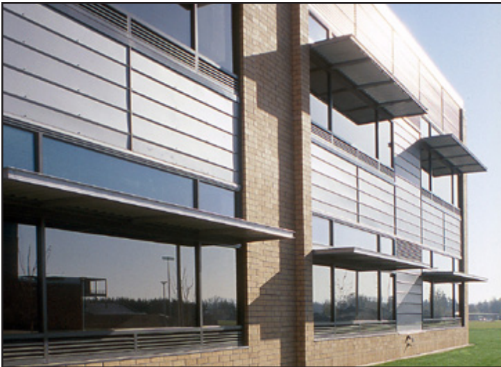
Sun Screens for Building Efficiency
